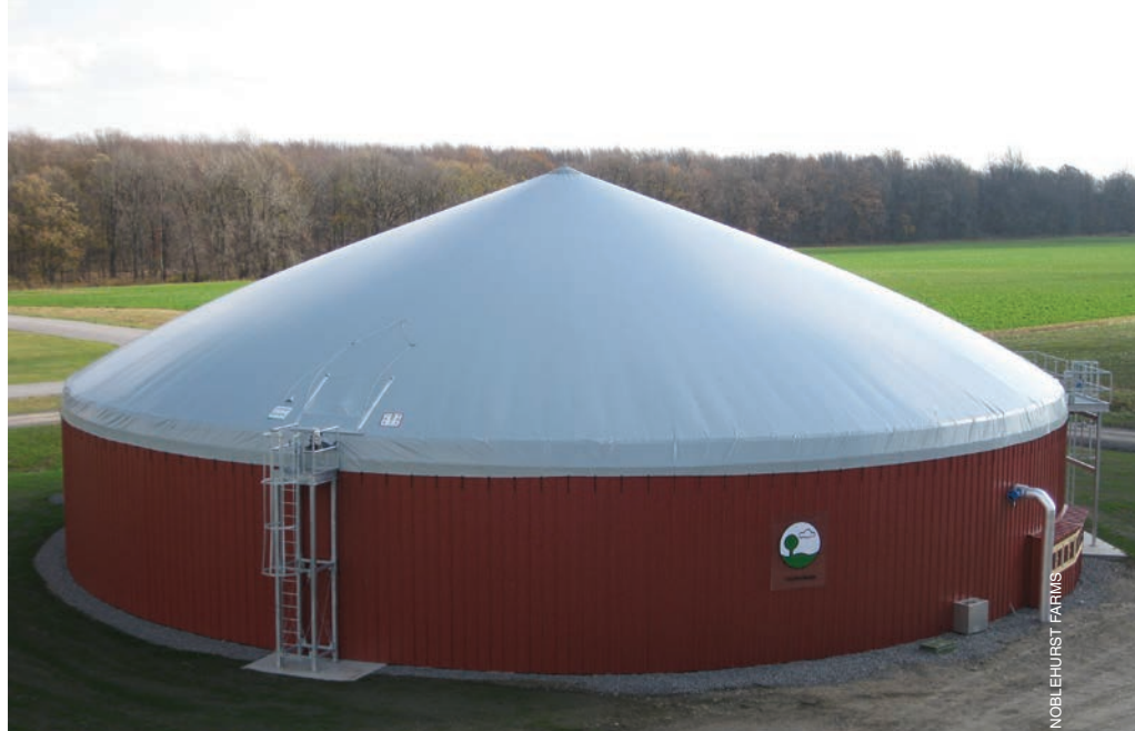
↗ Noblehurst Farms' anaerobic digester stores cow manure, and allows the farm to trap methane gas and use it to generate electricity.
